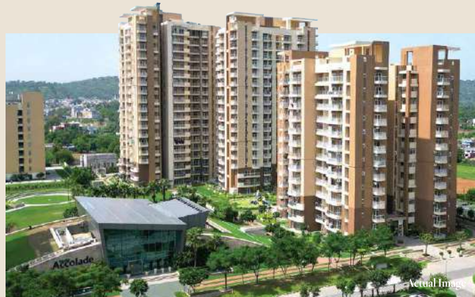
Eldeco Accolade, Sec 2, Sohna Road, Sohna
